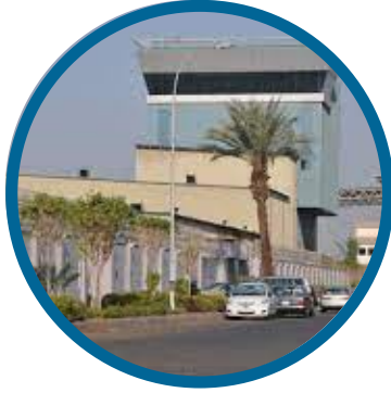
Jeddah Cables Company
